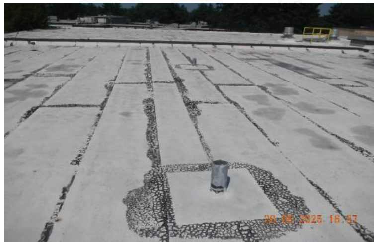
Photo 11 – Typical lead flashed pipe penetration.
