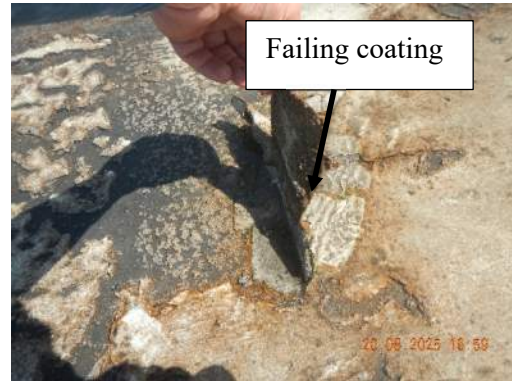
Photo 6 – Failing coating in ponding locations. The submerged coating material is separating from the cap sheet.
