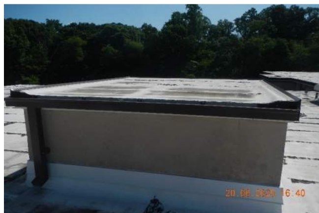
Photo 14 – Overview of penthouse gutter edge and downspout.
