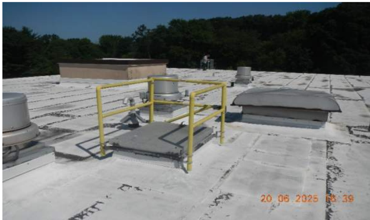
Photo 13 – Overview of typical rooftop units and penthouse roof section.
