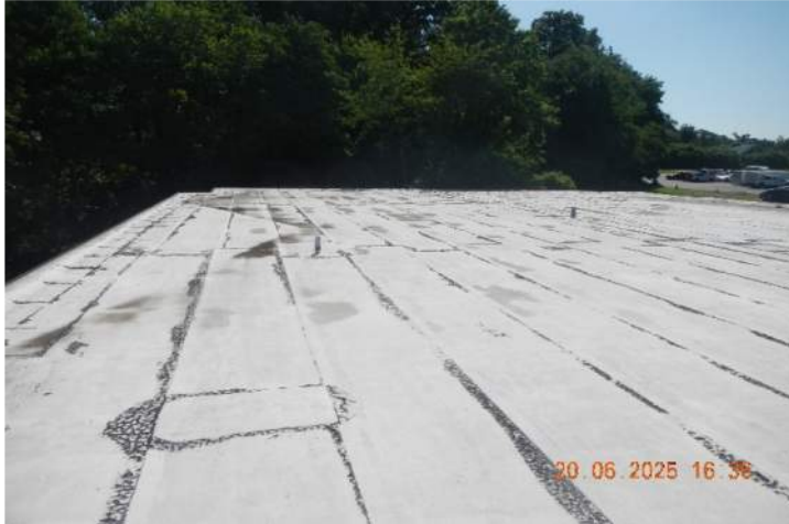
Photo 1 – Overview of upper roof section
