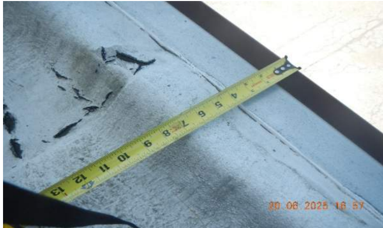
Photo 15 – Typical roof edge
