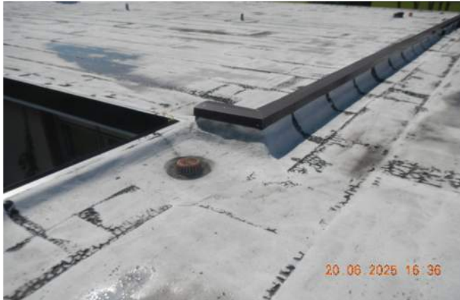
Photo 12 – Typical roof drain and roof divider.
